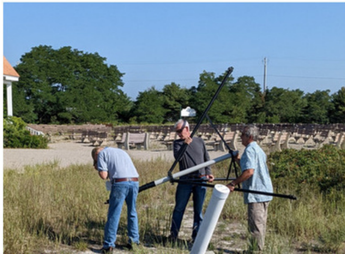
Dave-AA1LO, Jimmie-KC1ETT, and Rick-KB1ASM start the process of erecting the antenna.
